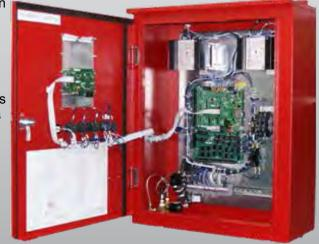
Controllers are completely wired, assembled, and tested at the factory before shipment and ready for immediate installation.
